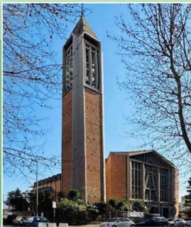
Exterior of S. Frances Xavier Cabrini Church
